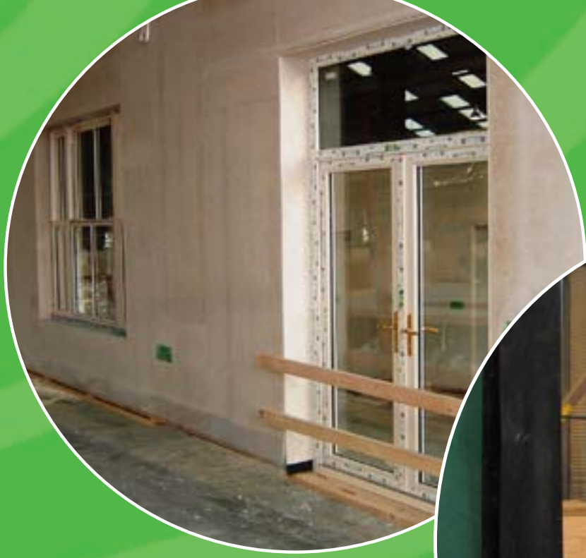
5. French doors fitted and sealed into a panel.
